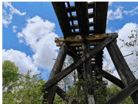
Figure 3.8 View under structure ID 1020201
