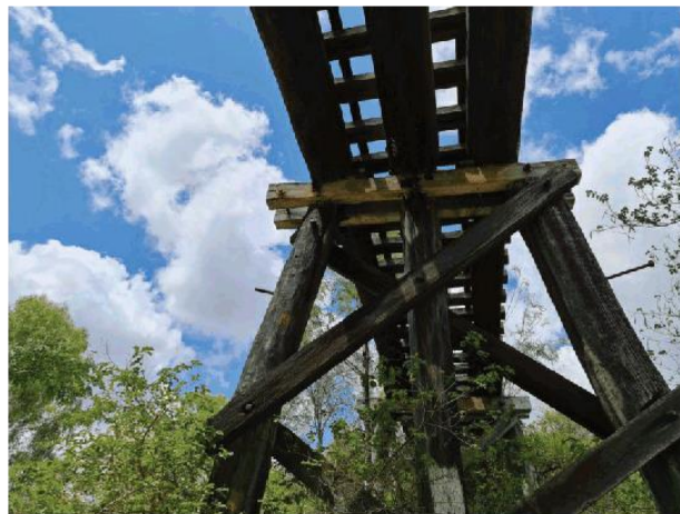
View of typical superstructure and substructure
