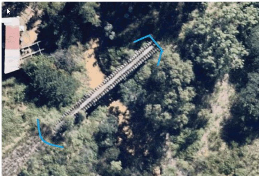
Figure 3.9 Illustration of permanent barrier blocking entry to Structure ID 1020200
