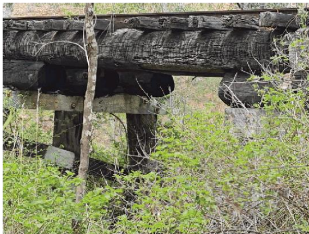
View of typical superstructure and substructure
