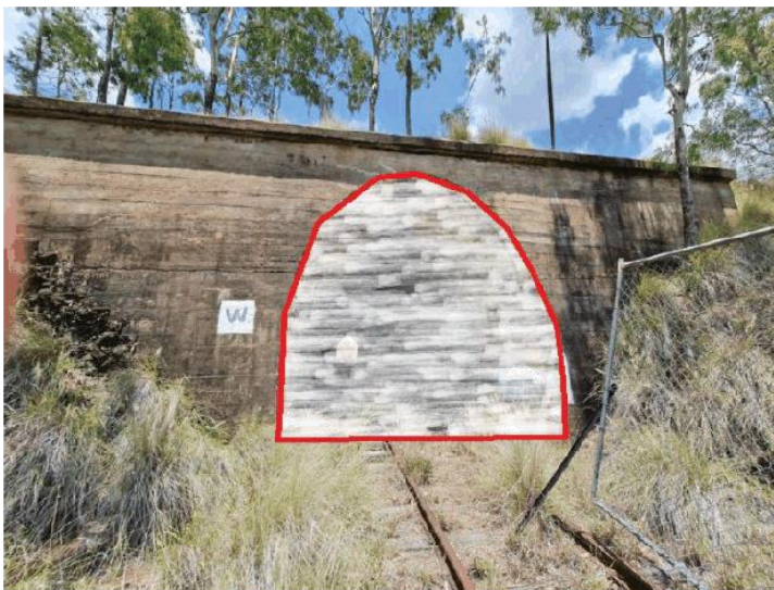
Figure 3.6 Illustration of permanent barrier blocking entry to Structure ID 1020200
