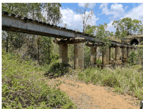
Figure 3.1 View of left hand side elevation of structure ID 1020199
