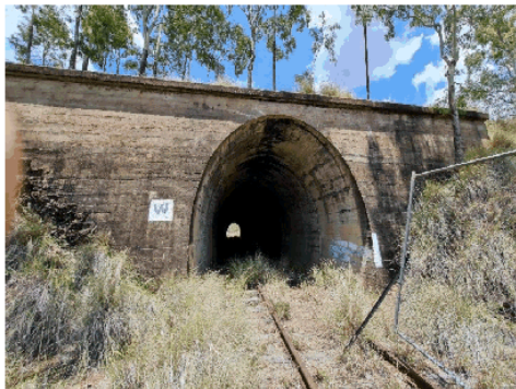
Figure 3.4 View of left hand side elevation of structure ID 1020200
