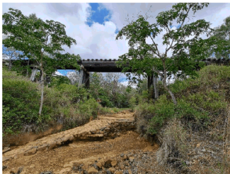
Figure 3.7 View of left hand side elevation of structure ID 10202001
