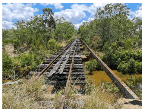
Figure 3.2 View from approach 1 of structure ID 1020199
