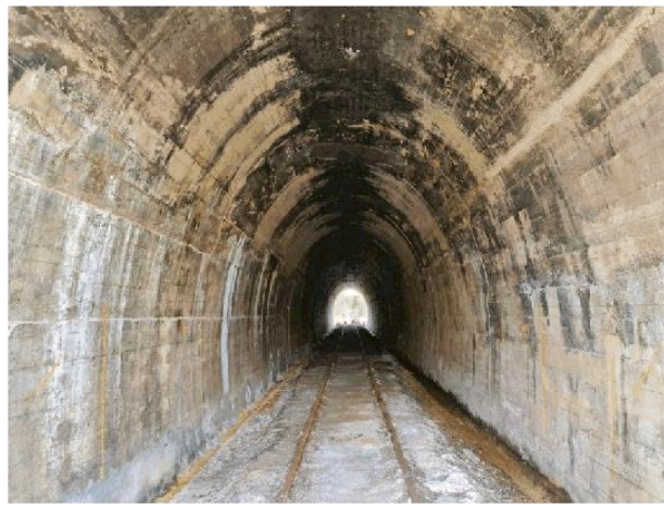
View of typical superstructure and substructure
