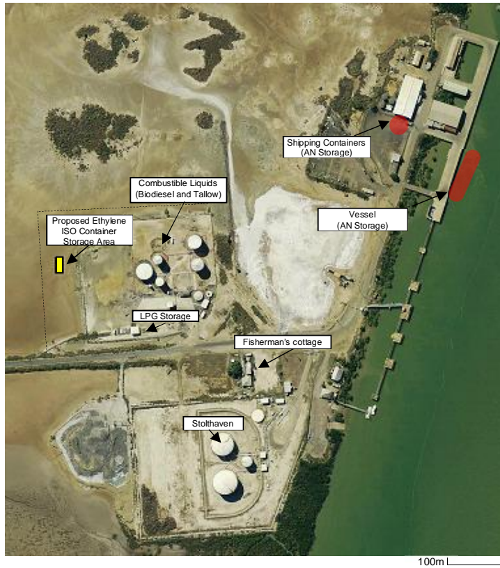
Figure 3 Portside storage facility, Lot 46 Bajool-Port Alma Rd, Port Alma, QLD
