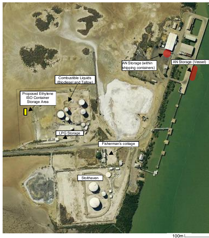
Figure 1 Portside storage facility, Lot 46 Bajool-Port Alma Rd, Port Alma, QLD
