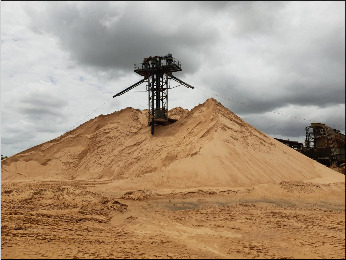
Figure 12. The Hydrocyclone and piles of recovered sand. The Hydrocyclone is the first stage of processing.
