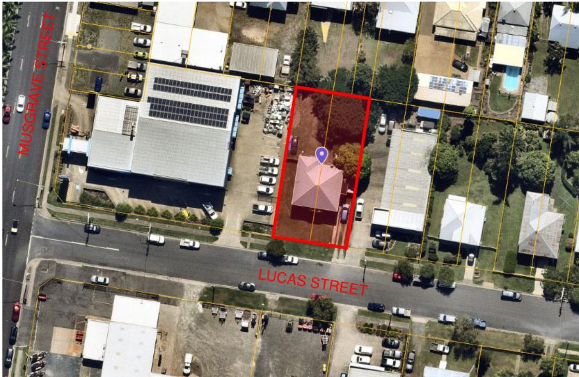
Figure 1 - 59 Lucas Street – Pre-developed Site
