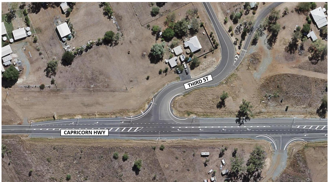
Figure 3-8: Capricorn Highway / Third Street intersection
