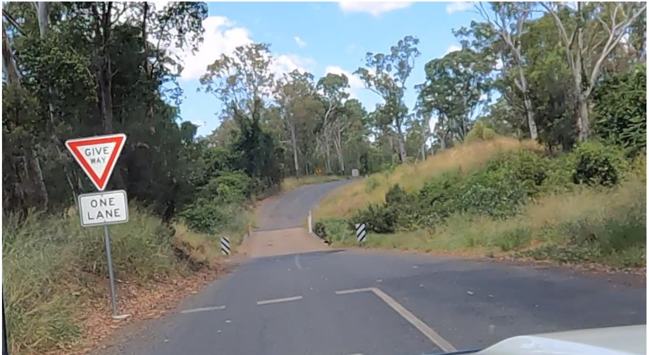
Figure 8-8: Floodway (Ch 2.9km) looking south from Give Way location
