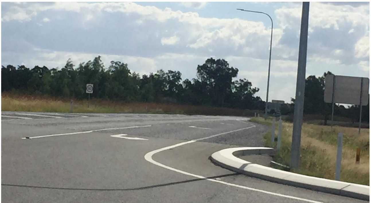
Figure 8-6: Available sight (looking west along Capricorn Highway from Third Street)
