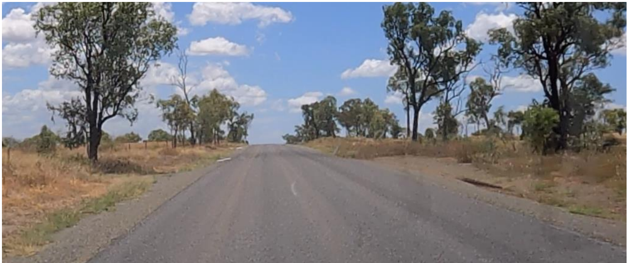
Figure 3-5: Thirsty Creek Road looking north (north of site access)
