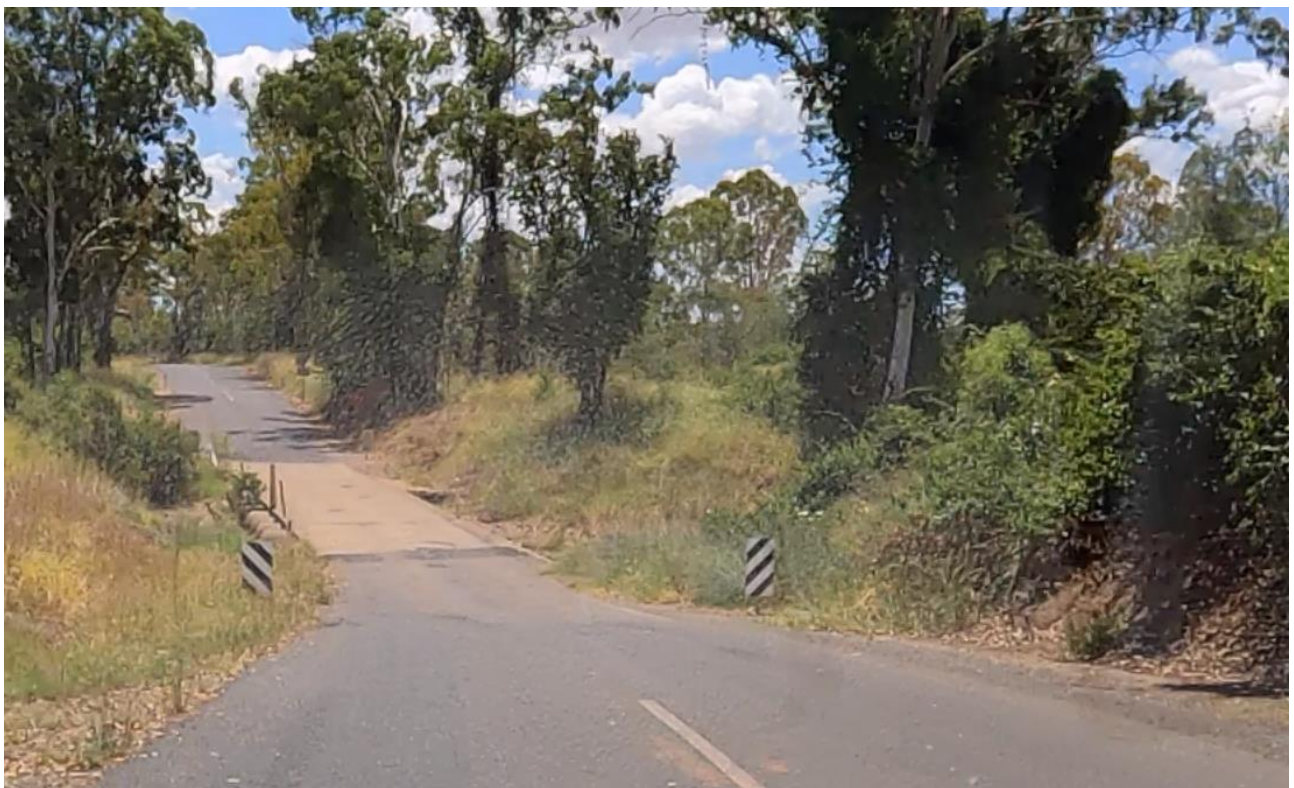
Figure 8-9: Floodway (Ch 2.9km) looking north from end of two lane section
