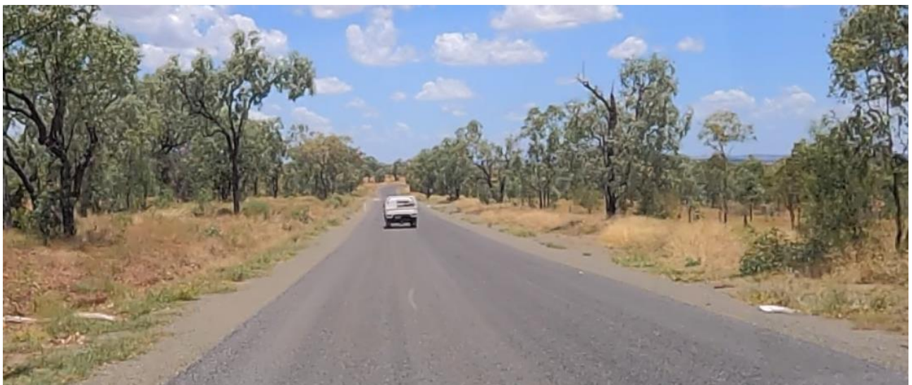
Figure 3-6: Thirsty Creek Road looking south (south of site access)
