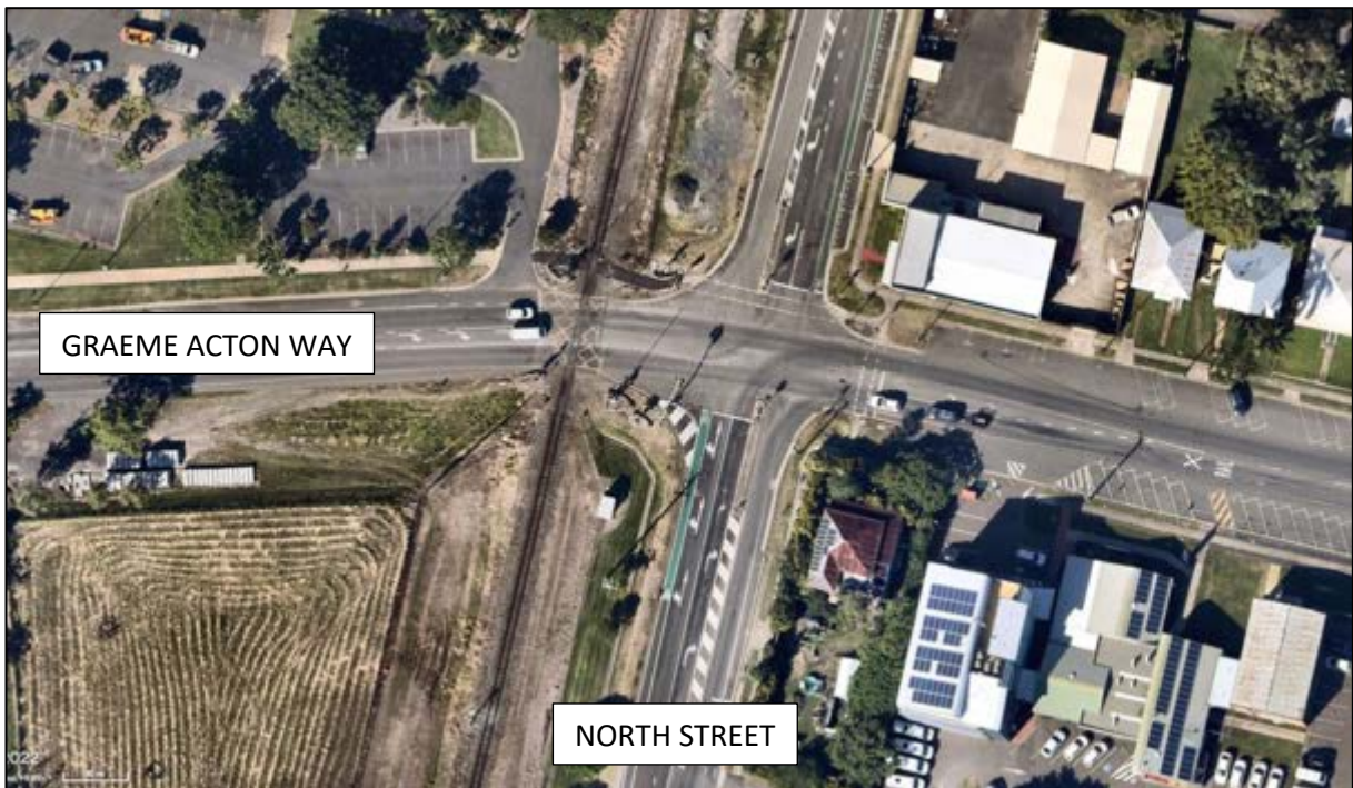
FIGURE 3.6 – AERIAL VIEW OF THE GRAEME ACTON WAY / NORTH STREET INTERSECTION
