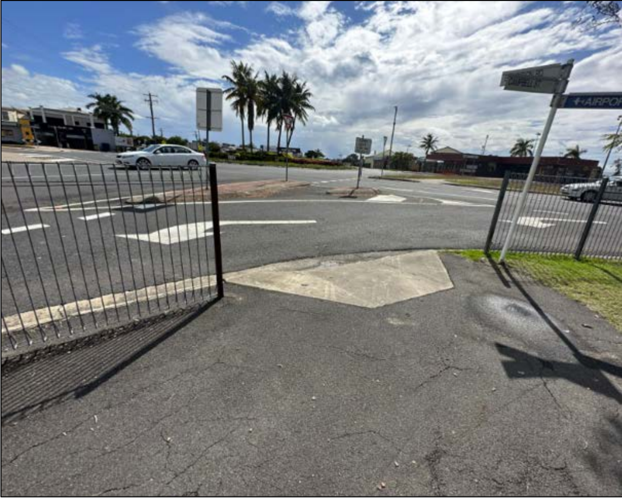
FIGURE 9.2 – IMAGES OF THE PEDESTRIAN FACILITIES ALONG CAMPBELL STREET
