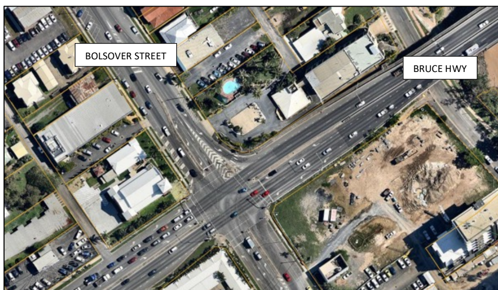
Bruce Hwy / Bolsover Street intersection
