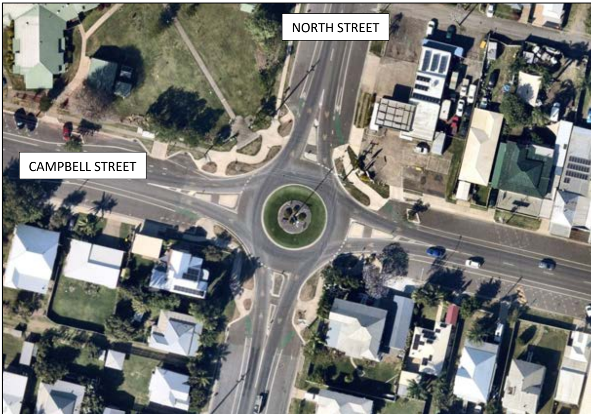
FIGURE 3.7 – AERIAL VIEW OF THE CAMPBELL STREET / NORTH STREET INTERSECTION
