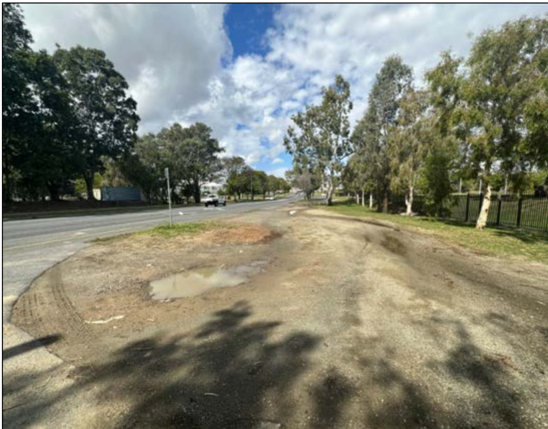
FIGURE 5.1 – PARKING VERGE ALONG GRAEME ACTON WAY
