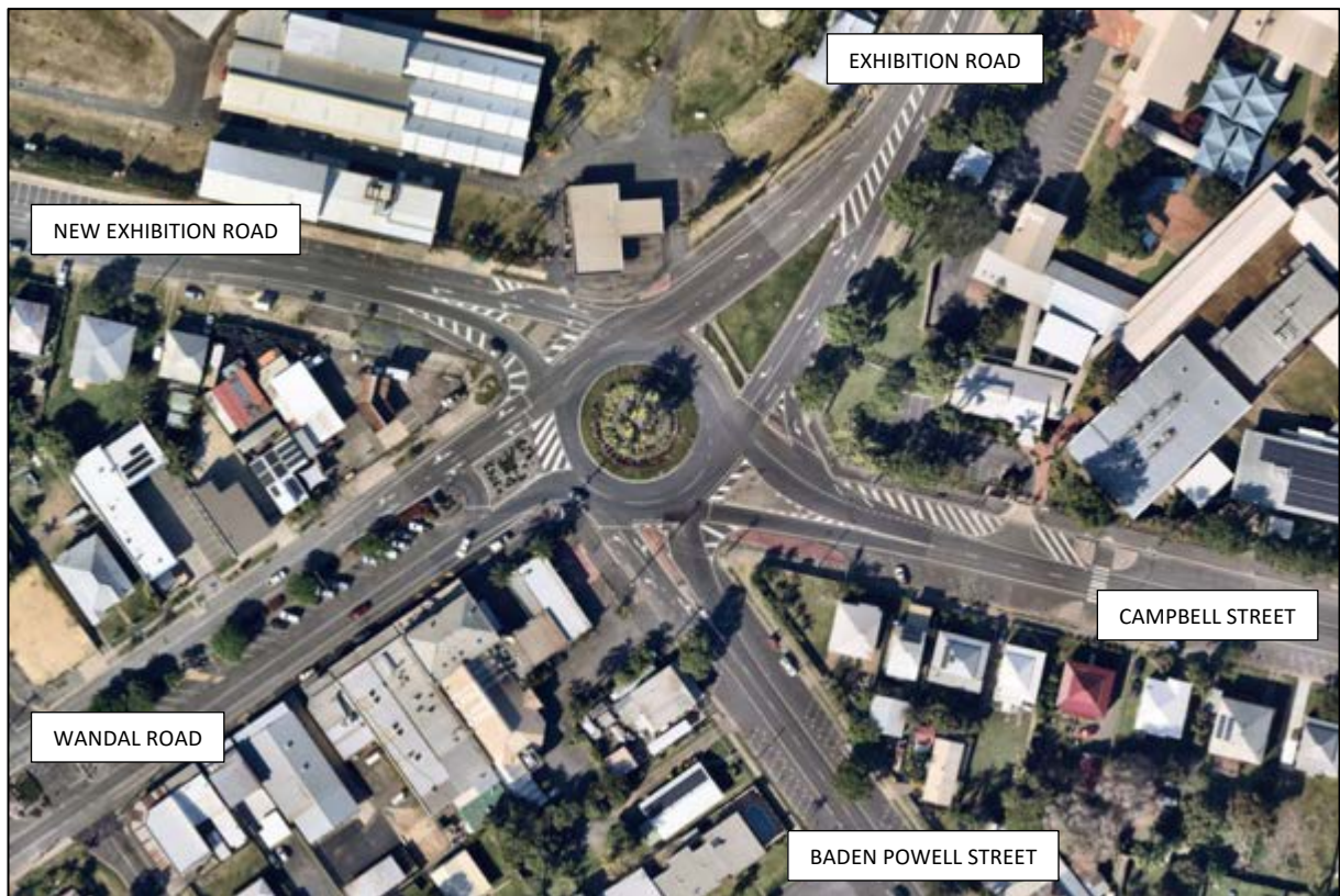
FIGURE 3.8 – AERIAL VIEW OF THE CAMPBELL STREET / WANDAL ROAD / BADEN POWELL STREET / NEW EXHIBITION ROAD / EXHIBITION ROAD ROUNDABOUT
