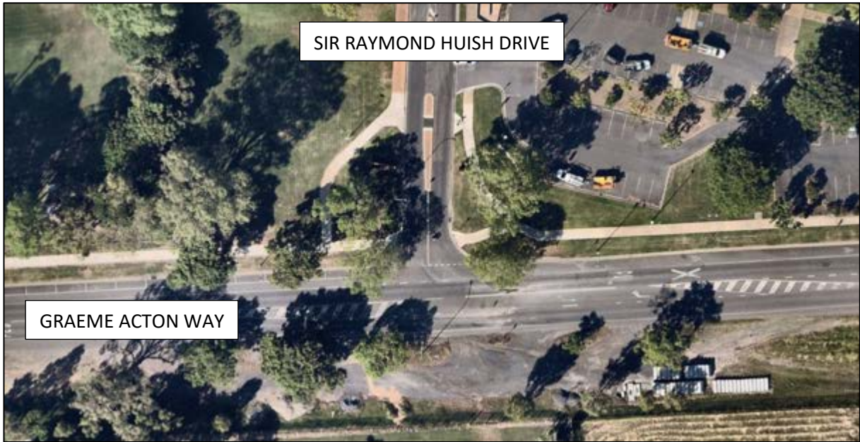
FIGURE 3.5 – AERIAL VIEW OF THE GRAEME ACTON WAY / SIR RAYMOND HUISH DRIVE INTERSECTION
