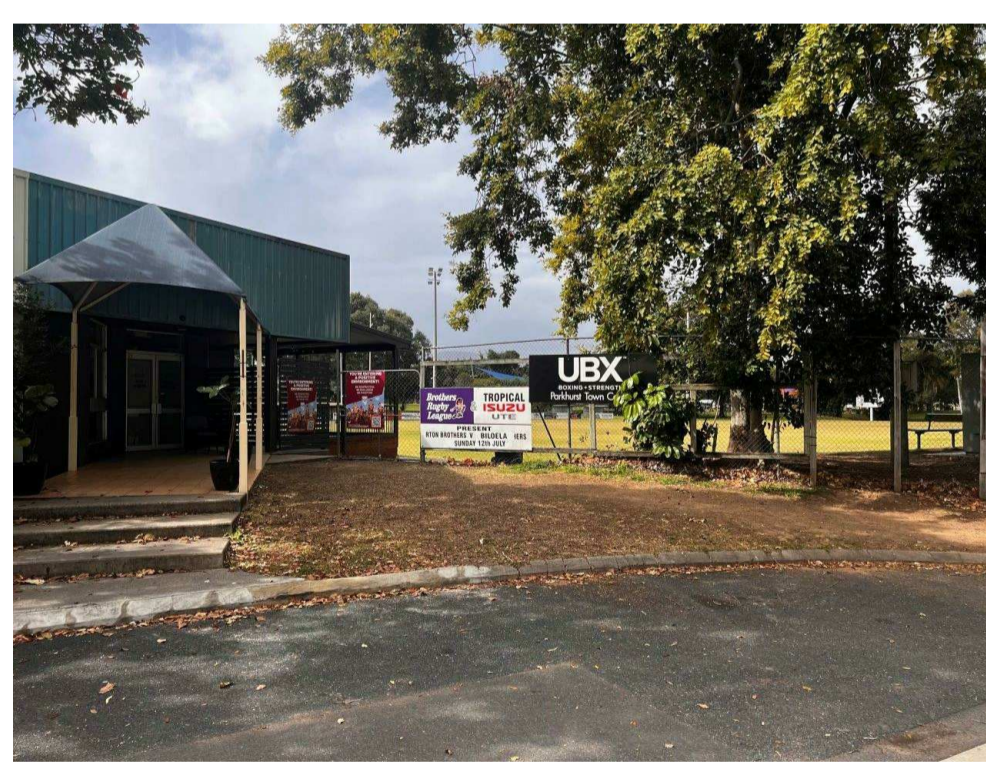
EXISTING CONDITION - PHOTO 1
