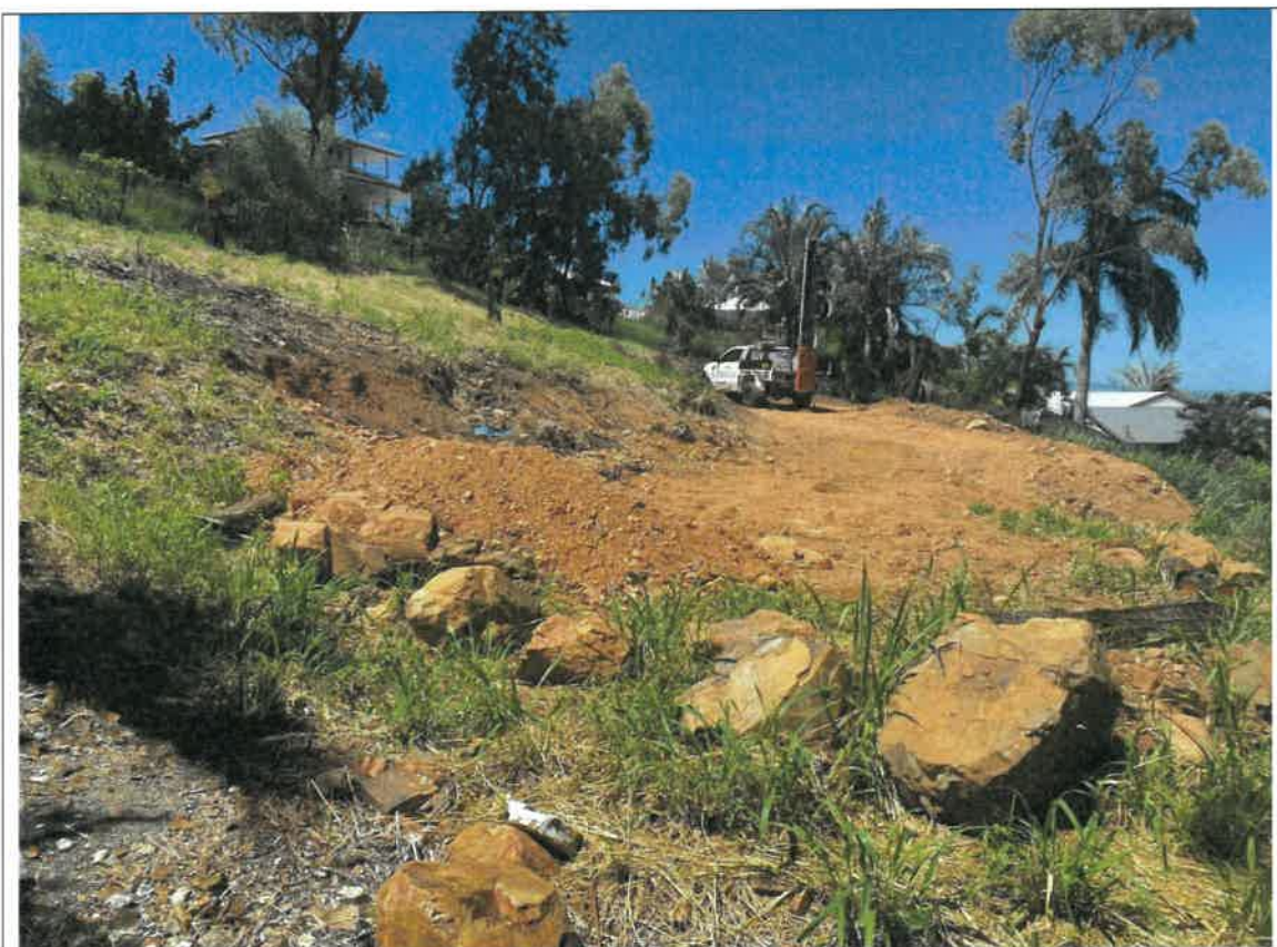
Image 4: Proposed Construction Site
