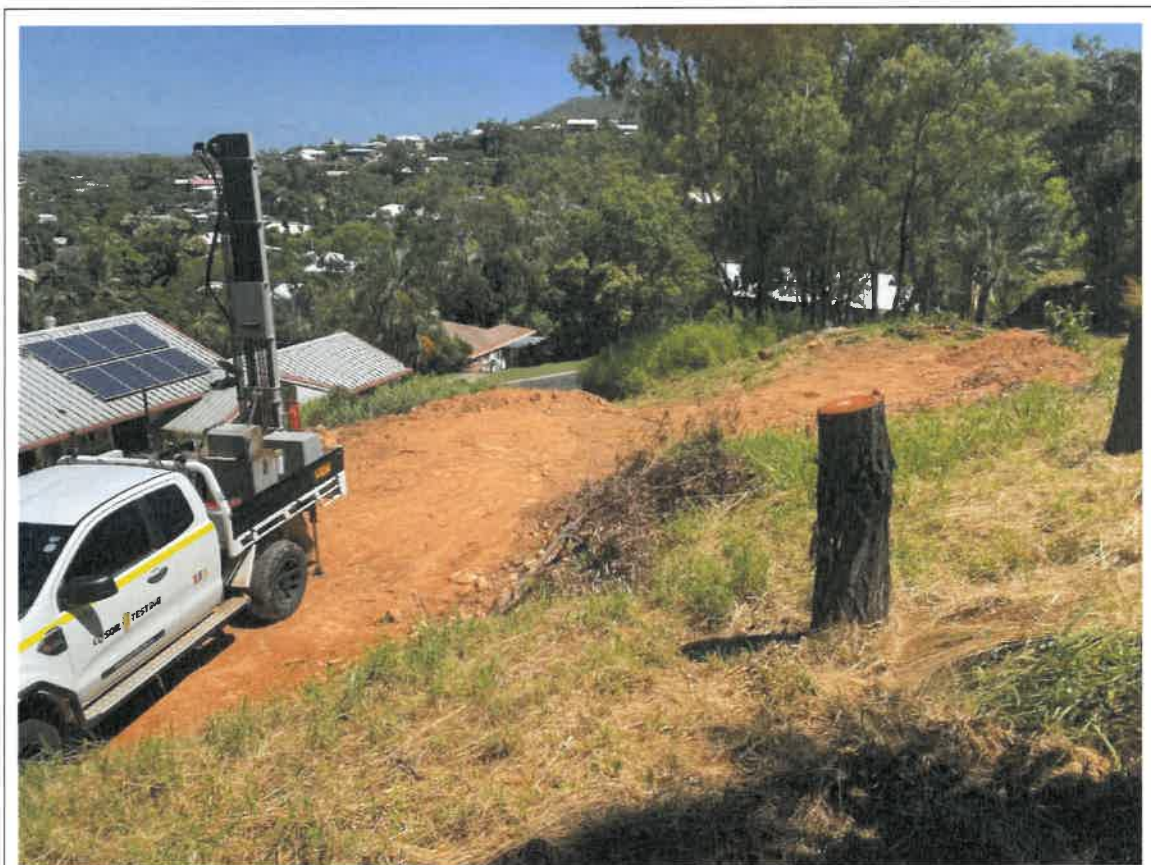
Image 2: Proposed Construction Site
