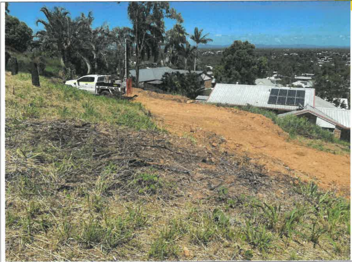
Image 3: Proposed Construction Site
