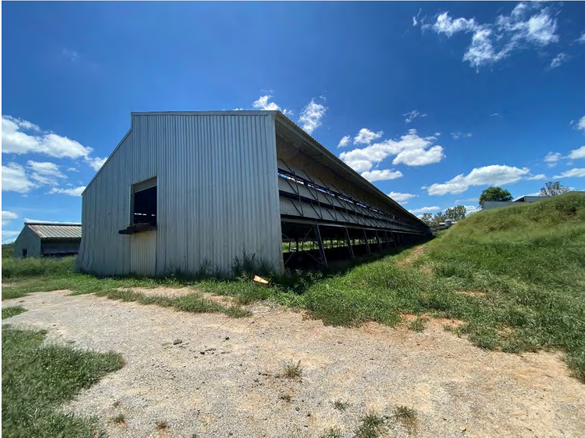
Photograph 1 – Existing sheds on the site
