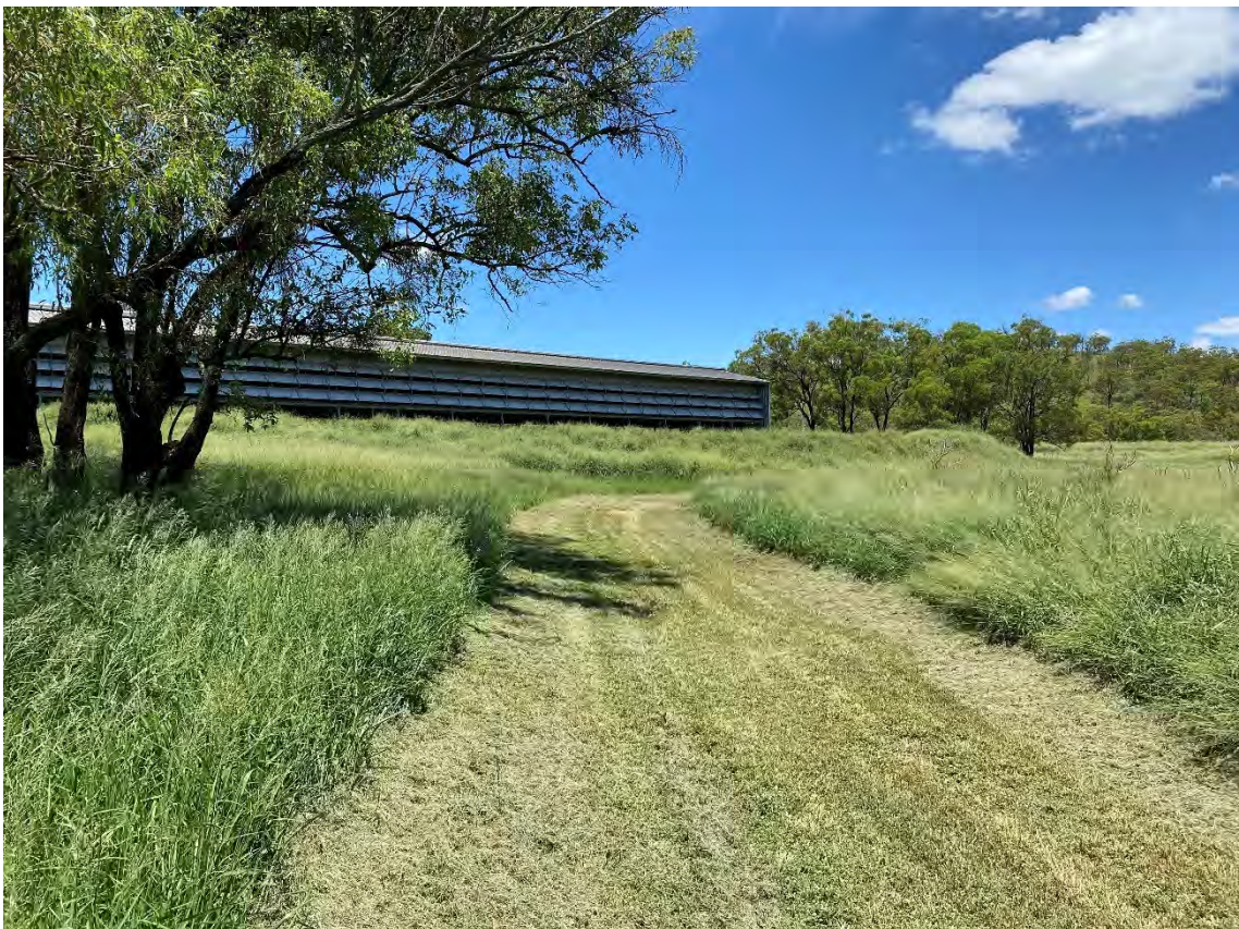
Photograph 2 – Existing site condition at the location of proposed Shed 4
