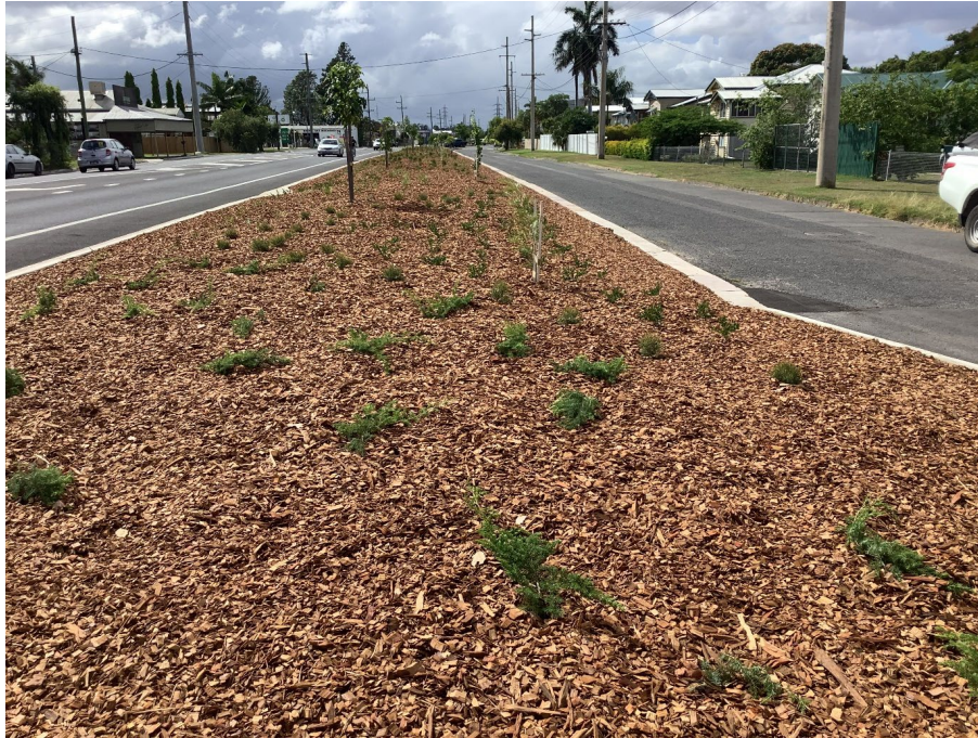
Glenmore Road median renovation
