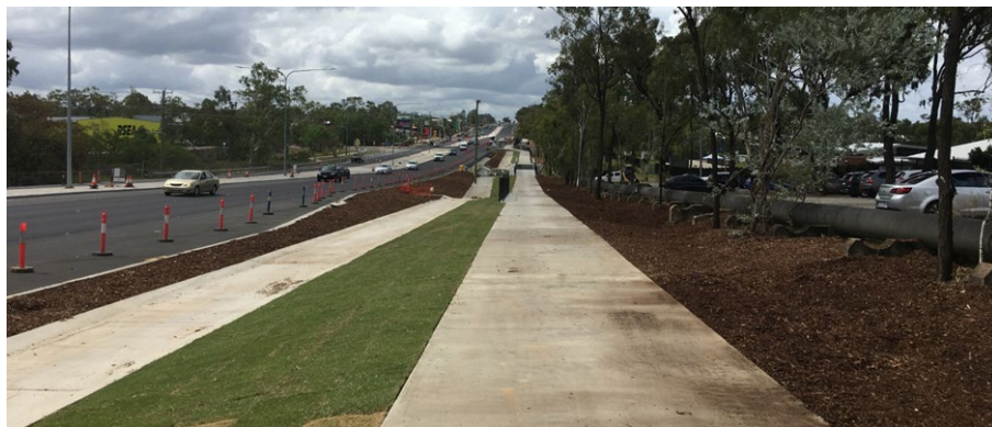
TMR works between Farm and Carlton Street
