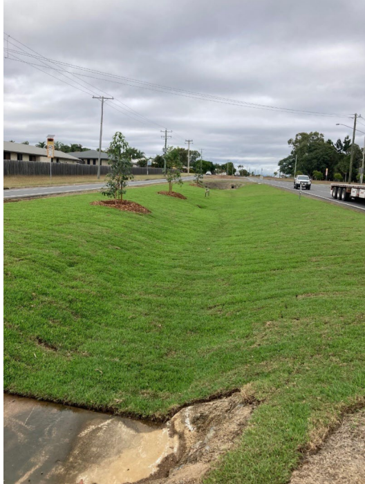
Johnson Road, Gracemere tree planting, civil works and irrigation completed.
