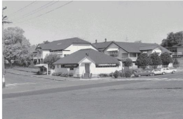
Figure 7: Commonwealth Bank, 1989 (SIQ Negative 201658)
