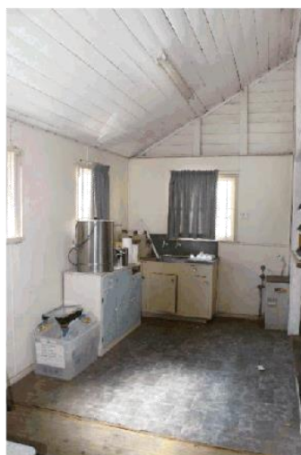
Figure 18: Enclosed verandah / kitchenette (AHS 2016)
