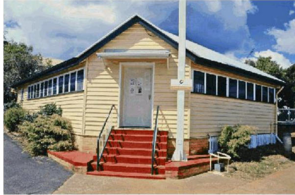
Figure 9: Commonwealth Bank Building, 2001 (QHR)
