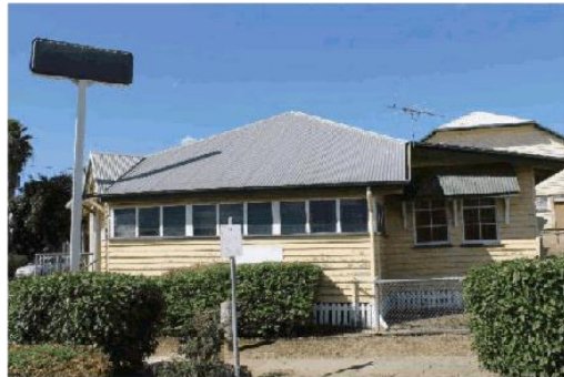
Figure 11: Building from Central Street, showing enclosed verandah and skillion office extension (AHS 2016)
