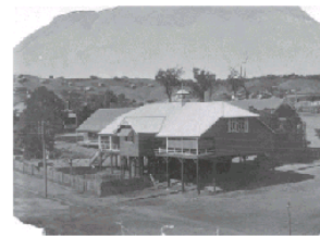
Figure 4: Mount Morgan State School Building, 1914 (SI Q Negative 1914)
