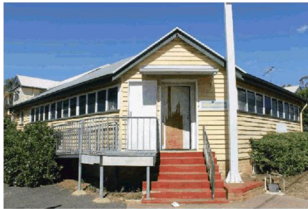
Figure 10: Commonwealth Bank Building, 2016 (A115)
