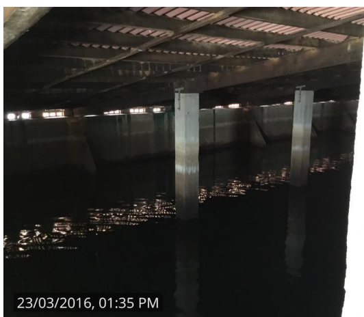
Internal view of original reservoir
