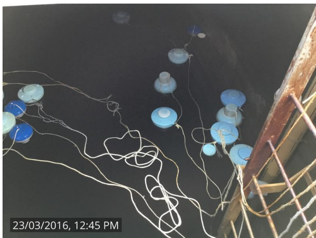
Floating chlorine tablets
