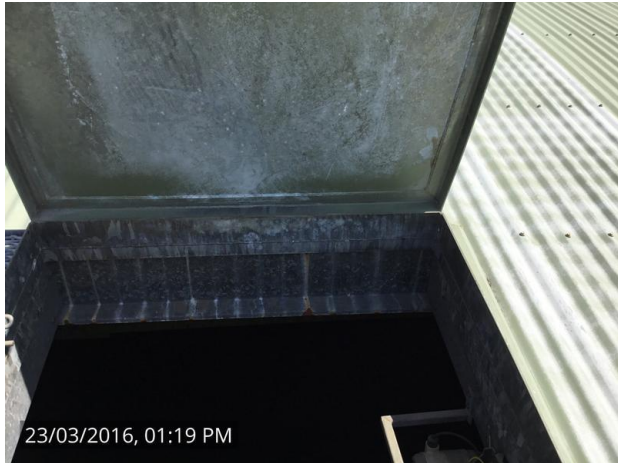
Athelstane B Hatch – close fitting, no other seal necessary
