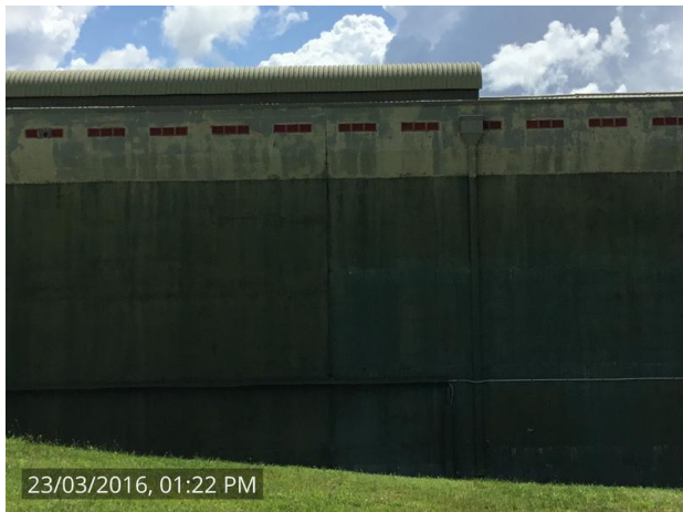
Original Athelstane reservoir – note the terracotta air vents
