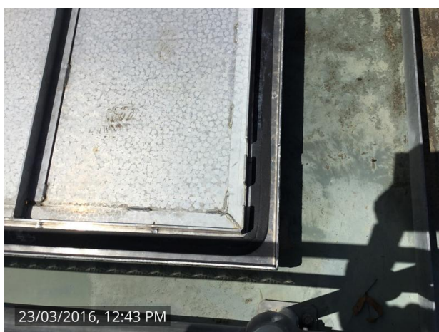
Rogar reservoir hatch – note seal in excellent condition
