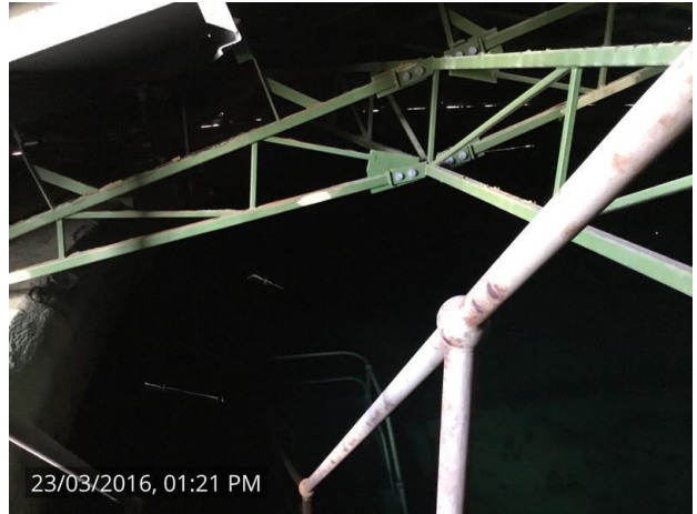
Internal view, ground level reservoirs
