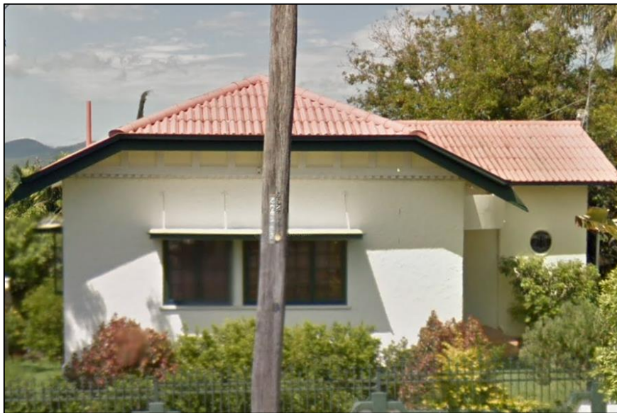
February 2015 street view – tiled roof, hipped roof evidence above gable frieze
