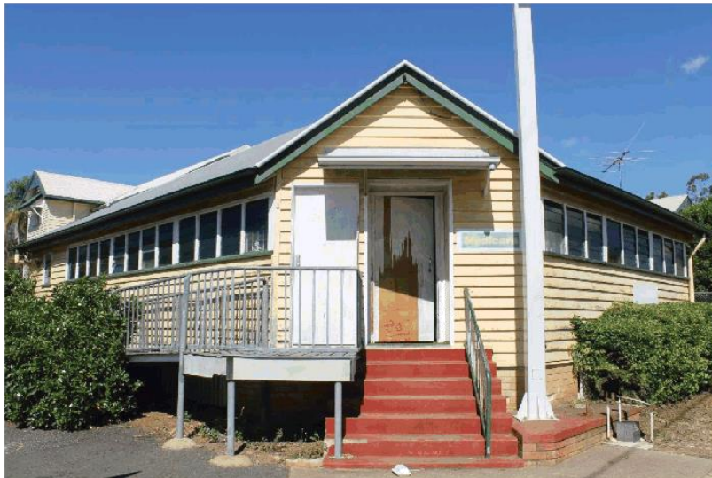
Figure 10: Commonwealth Bank Building, 2016 (AHS)
