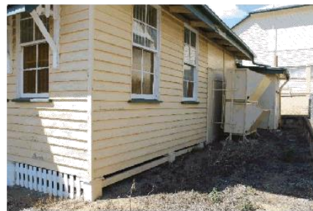
Figure 13: Skillion office windows (west) - (AHS 2016)
