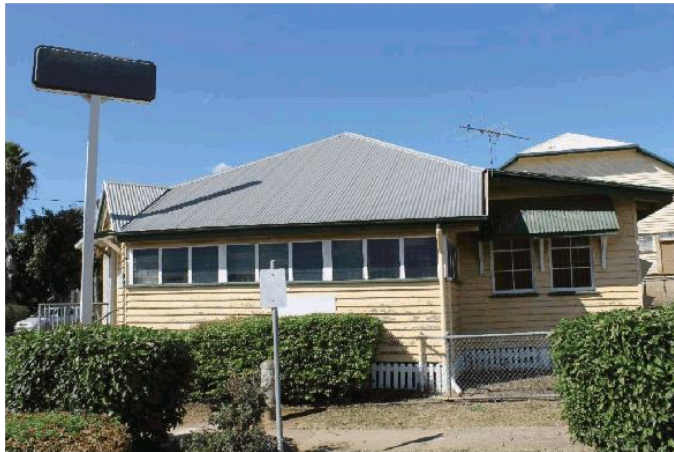
Figure 11: Building from Central Street, showing enclosed verandah and skillion office extension (AHS 2016)
