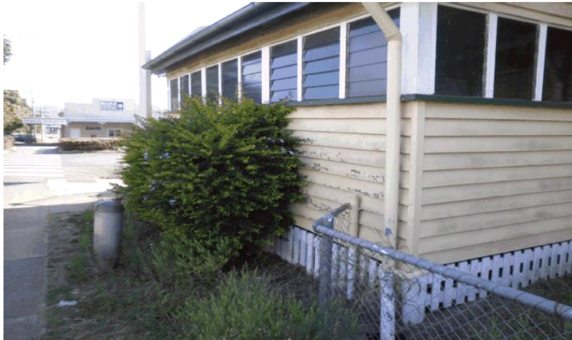
Scrubs against western side of the building. (Photo 3)
