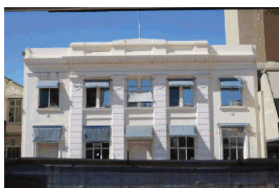
Figure 25: Commonwealth Bank of Australia (former) Townsville
