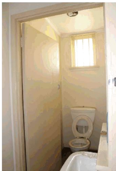
Figure 19: Toilet under skillion (AHS 2016)
